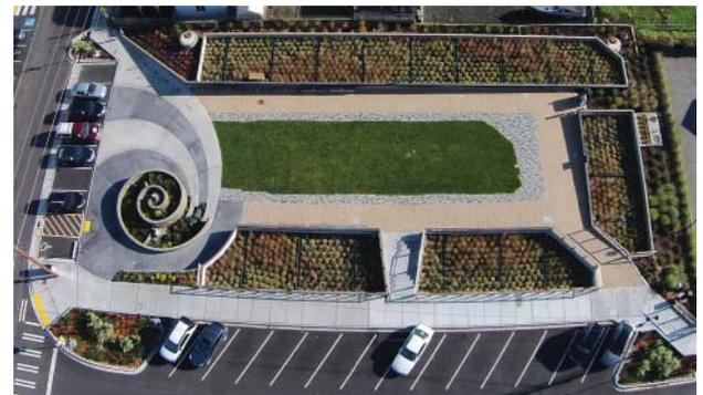
After construction: the four treatment cells contain filter media and plants to clean the runoff before it reaches Puget Sound.
