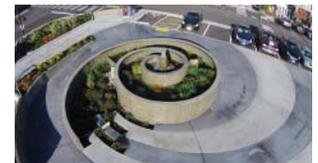
The spiral rain garden is not only aesthetically pleasing but is designed to treat low flows from groundwater and small storms to assist the larger treatment cells.
